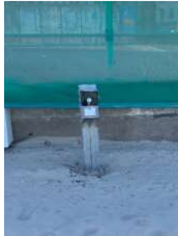
Tap 5 – Opposite 2 nd Bus Shelter
